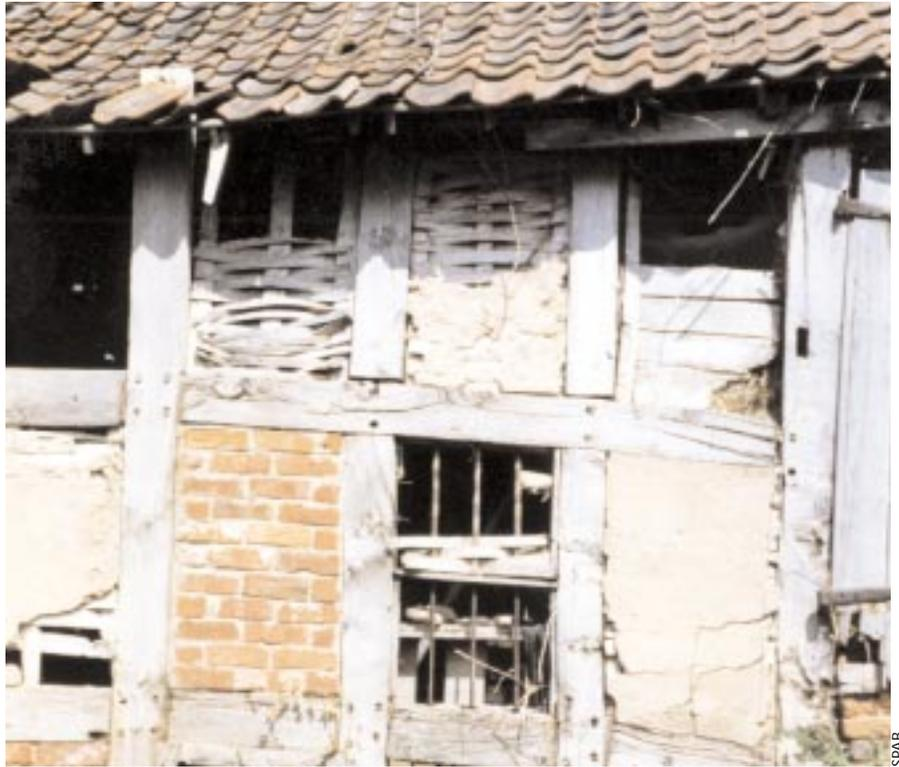
A decayed timber framed wall with infill panels of original wattle and daub and later brick
