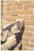
If you are chopping out failed or cement pointing, make sure that the chisel is narrower than the width of the joint, so that the edge of the brick does not get damaged
