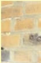
Inappropriate and unnecessary repointing carried out in cement. The original penmanship pointing is shown to the left
