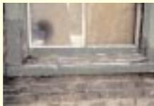
A cill and window now decaying because of missing paint and putty
