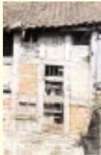
Detail of a timber-framed building, showing movement in the frame, deterioration of the brick infill panels and poor previous repairs
