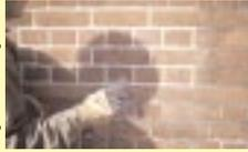
Hand-finishing new lime mortar pointing with a churn brush, to reveal aggregates and ensure that the arrises (edges) of the bricks are clearly defined
