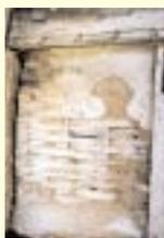
Lime-coated wattle and daub panelling is quite rare. Although poor maintenance has led to decay in this case, the damage can be repaired
