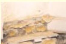
Dry rot is a symptom of water getting into the building, coupled with poor ventilation
