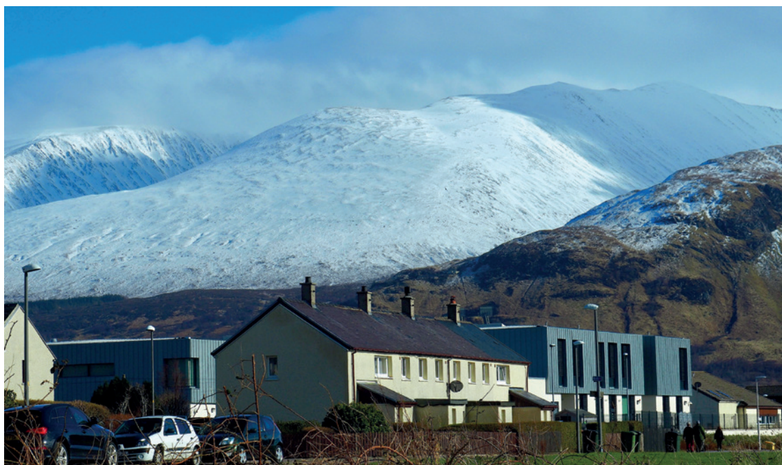
Upgrading the insulation in traditionally constructed buildings is now known to be a more effective way to meet the UK's 2050 net zero targets than demolition and renewal.
