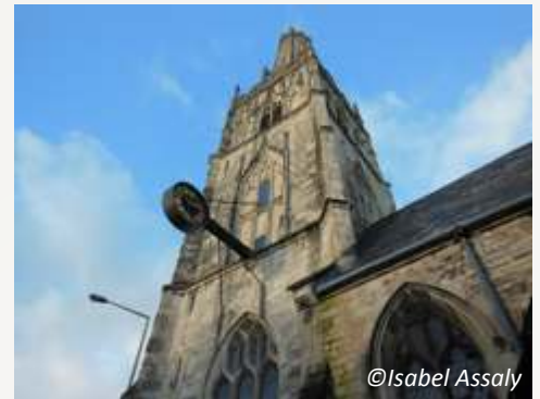
St Nicholas' Church on Westgate Street; the oddly truncated spire is the result of lowering/capping following damage sustained during the English Civil War siege of the city in 1643
