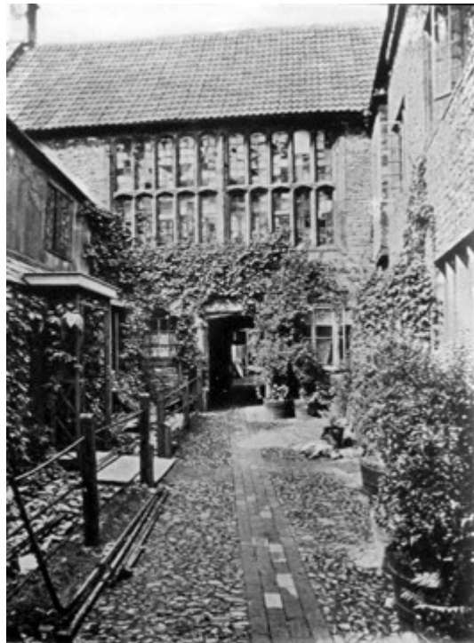
Pic 3. South elevation of Courtroom block circa 1900
