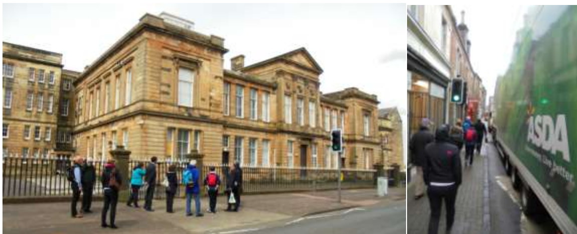
IHBC at former Ayr Academy and in Maybole, said to need a by-pass (©Mark Watson)
