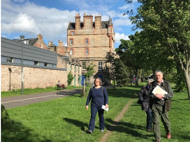
New and old at a development by LDN at Archers Hall, and the converted Boroughloch Brewery, now a tenement. Photo: Mark Watson
