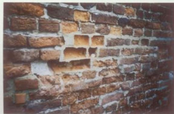
It should always be remembered that 'hard onto soft' will not work. Often one sees 'new' shallow pointing falling off the front of the joints. This is not only because it was shallow but in application the joint may not have been 'wetted in or cured' properly. Any mortar if cementitious or stronger it has a greater potential for shrinkage and is loosened on initial drying out. Pinch points can be caused with a hard mortar putting stress on the hard fired brick edges.
