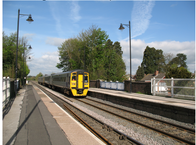
Site without the footbridge
