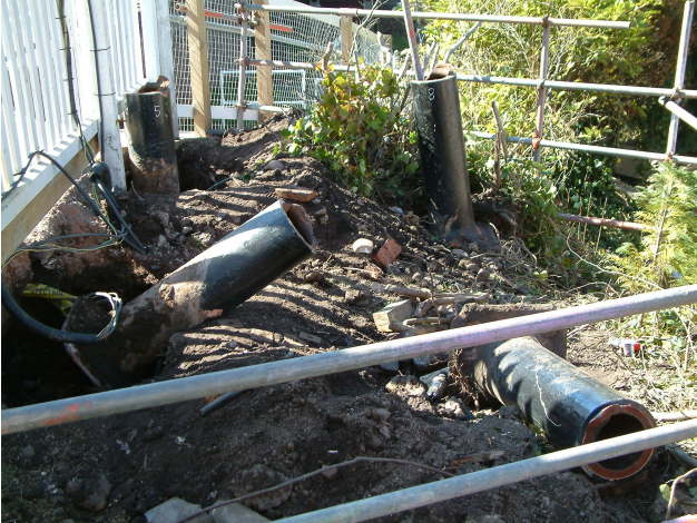
Original column bases in situ
