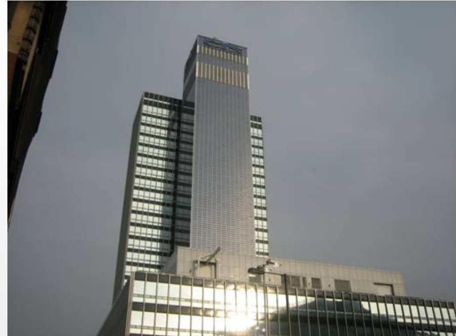
CIS Building, Manchester
