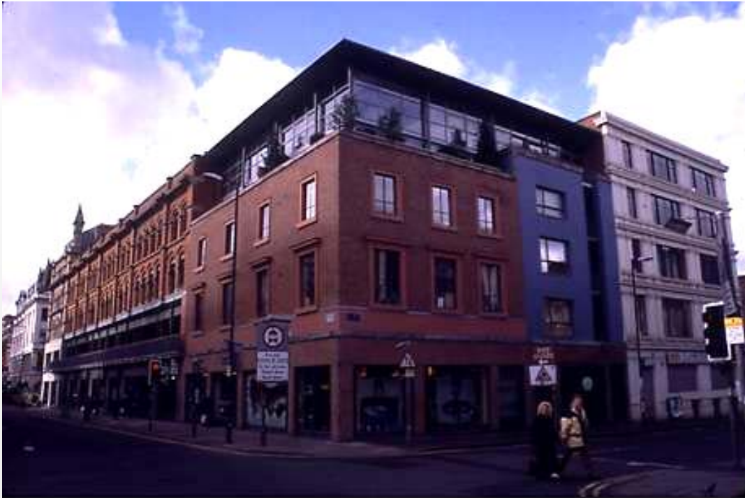
Mixed use building conversion, Manchester
