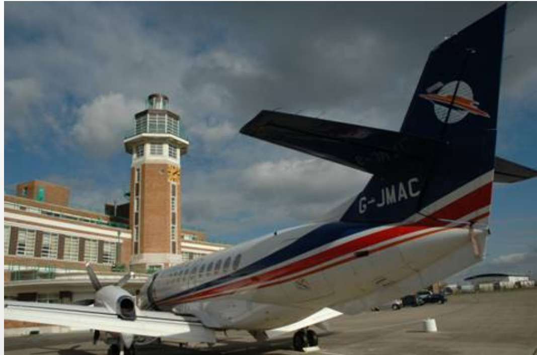
Former airport buildings, Speke, Liverpool
