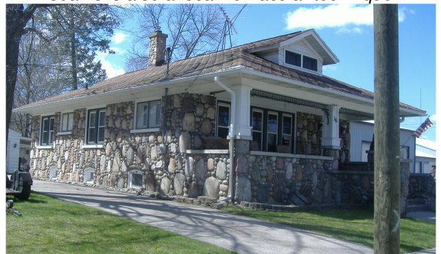
House in Saranac, Michigan, using alternating rough-dressed boulders and cobbles.
