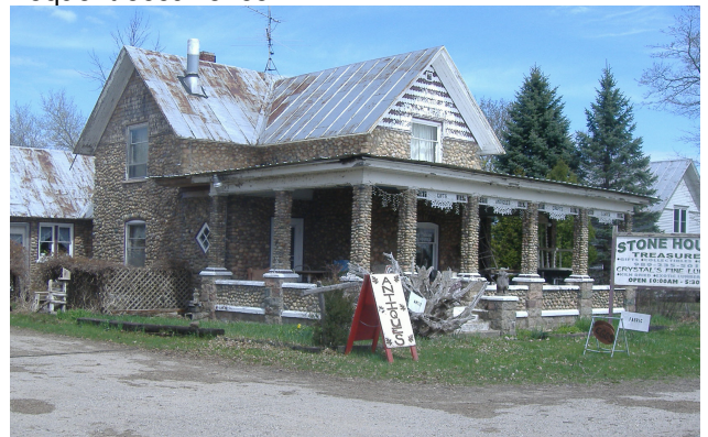
Vernacular cobblestone-built house in Crystal, Michigan. Tin-plated sheet metal roof with raised seams is also a local vernacular technique
