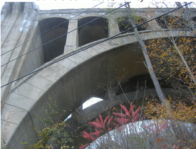
Martin's Creek Viaduct. Detail, showing frost damage high up.
