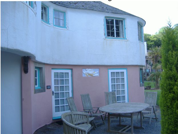
Fraying at the edges, with cracking render and rust stains from old steel frames
