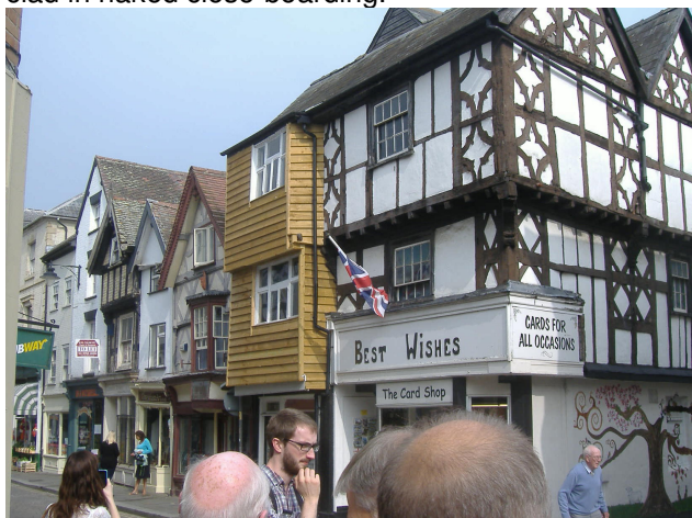
Unauthorized alteration. Close-boarded cladding added to jettied Listed Building
