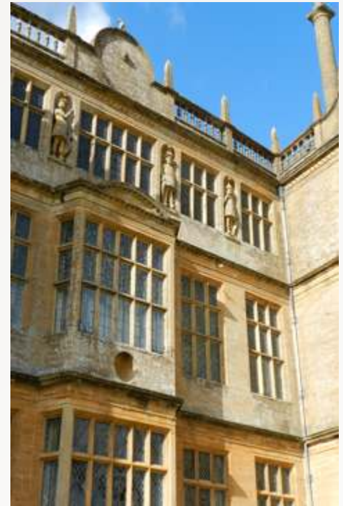
Part of the south front at Montacute showing the relatively large ratio of glazing to load bearing masonry; most notably to the top floor (housing part of the National Portrait Gallery)
