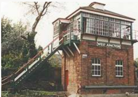
Bournemouth West Junction signal box dates from 1882 and is a good example of the LSWR 'type 3' structure with its tall elegant form and distinctive toplights above the horizontal sliding sashes (image © Alan Elliott 1992)
