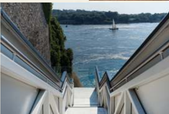
Clockwise from top-left: View of staircase providing a link between the green space beyond the high retaining wall (right) and the Royal William Yard (left) with Devonport beyond; staircase at night showing integral lighting; view west over Tamar Estuary to Mount Edgcombe, Cornwall (images © Richard Downer)
