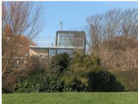
View of development from Old Castle Road (top) and the "sculptural form" of the extension as seen from Sandsfoot Gardens in 2010 (bottom)
