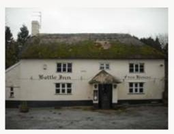
The Bottle Inn mid-2011 with deterioration of the thatched roof coverings visibly apparent
