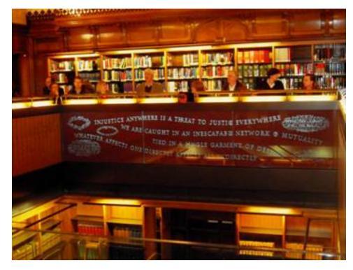
In some areas, the use of some heavy-duty quite secondary glazing apparent. was This unfortunately intrusive feature was necessary, for both sound reduction and because of potential security threats. In contrast. the glazing over of a light well within the building, not created only additional useable space, but also
